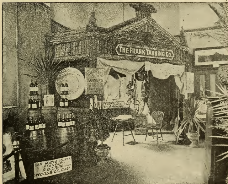
SAN MATEO COUNTY BUILDING—INTERIOR
